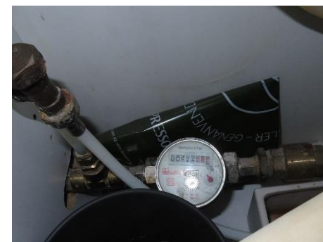
Messingfitting i rustfri installation
